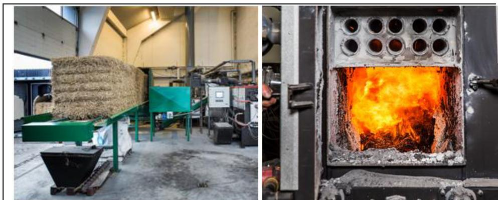
**Figure 1** - Combustion equipment: feeding 200 Kg straw bale (right) and burning in the boiler (left)
